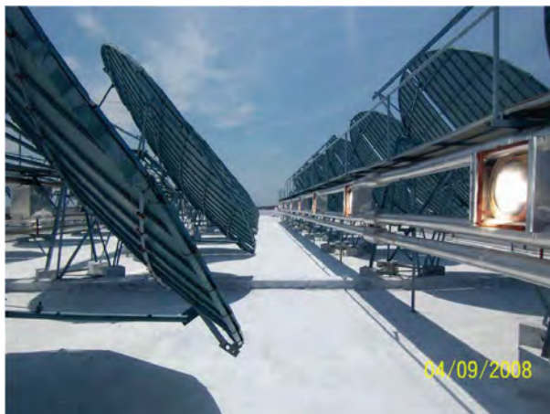
Scheffler Parabolic dishes generating heat at 140 °C
