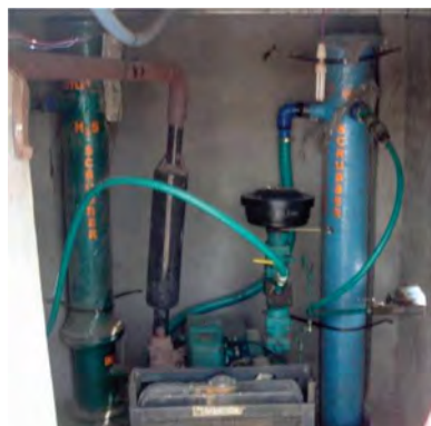
Gas Engine for m 3 biogas digester
