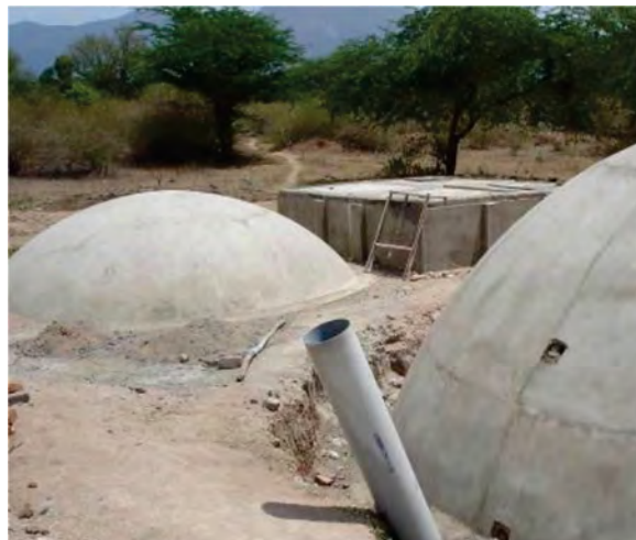
65 and 35 m 3 biogas digester
