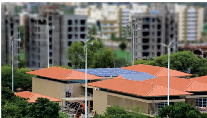
Aerial view of Renewable Energy Systems installed at Suzlon
